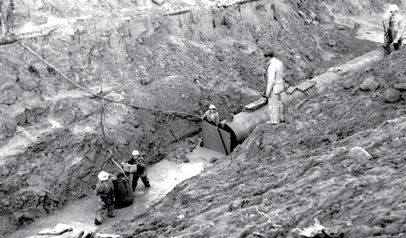
MEGAPROJECT FOR MEGAWATER: 1960 construction of the concrete and fibreglass pipe carrying Haslam Lake water to the treatment plant.
