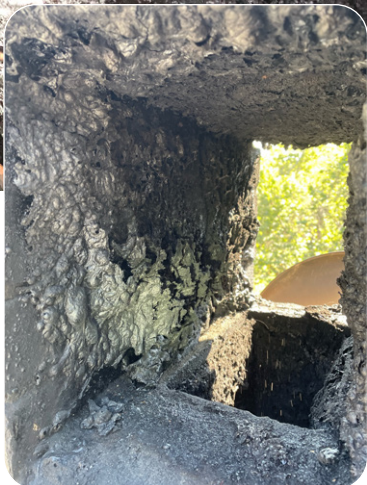
NOT YOU, WE HOPE: Top, a structure fire has reduced this house to ash. Right, this chimney is desperate for a cleaning.
