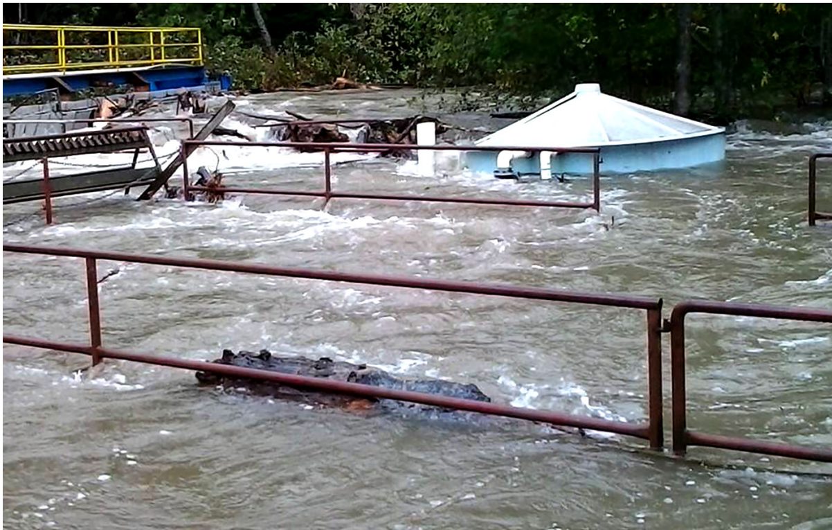
2014 VERSUS 2021: Flooding hit qathet harder in 2014 than it did in 2021. Here, the Tla'amin salmon hatchery was under water in 2014 – reducing salmon returns five years later. Photo courtesy of Tla'amin Nation
