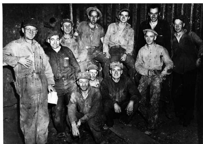
LIKE DANTE’S INFERNO: That’s how Dr. David May describes the hot, loud, physical environment at the mill when he first toured it 30 years ago. Above, the #7 boiler crew in 1947.
